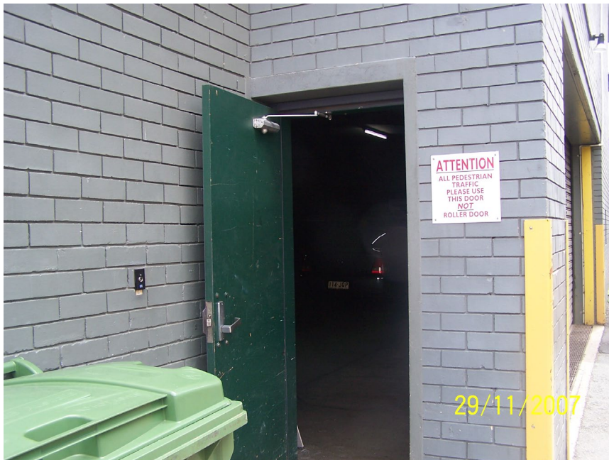
Level B - Photo No: 78 Access – Door (Fire)
