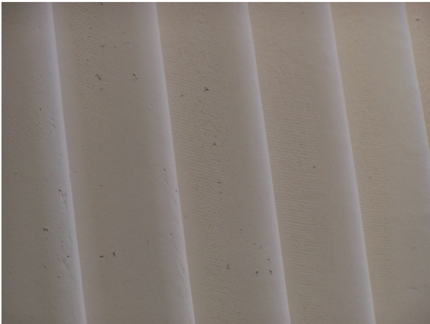
Photo No: 102 Exterior – Cladding
