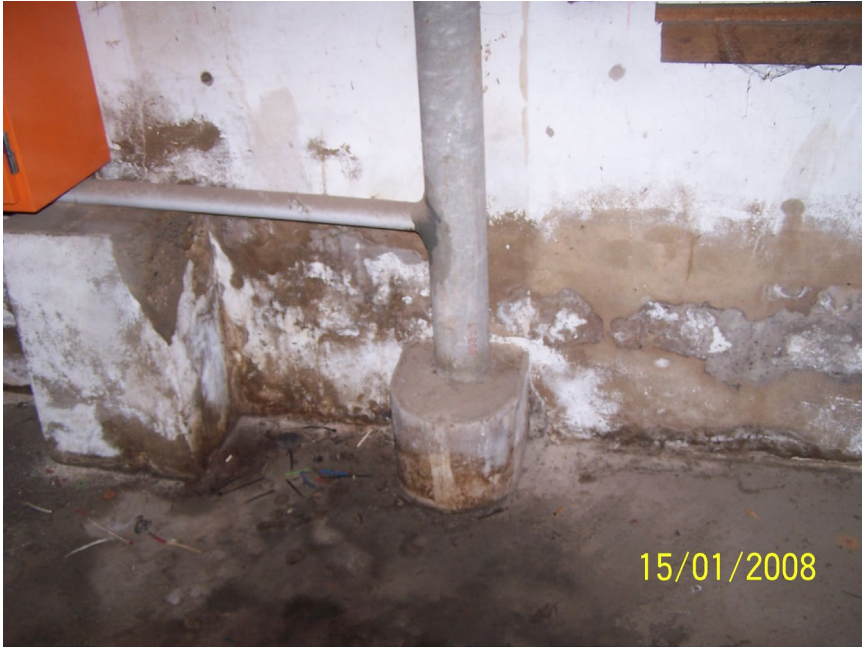
Photo No: 235 Unit 15 A Workshop – Org Surround
